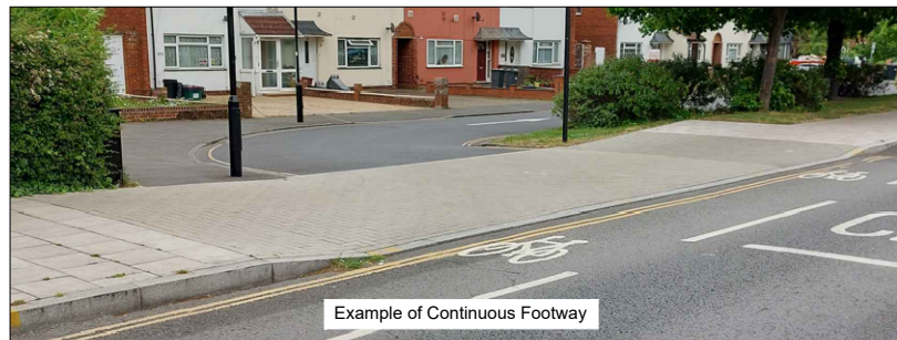
Typical Side Road Entry Treatment
